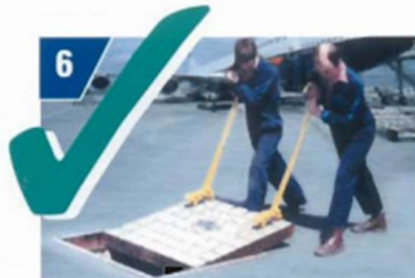
6 Turn the EZI-LIFT through 180° to slide the cover back into place to re seat
