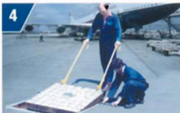
4 For extra large or very heavy covers, note the use of round bar to assist movement
