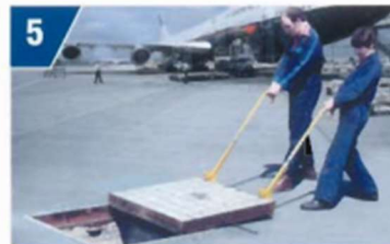
5 Cover can now be fully removed
