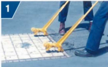
1 Use the EZI-LIFT inverted to break the seal of tight covers
