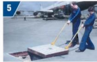
5 Cover can now be fully removed
