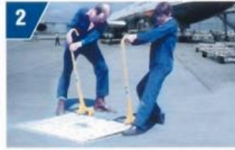
2 Gently pull back the EZI-LIFT's to raise one edge of the cover
